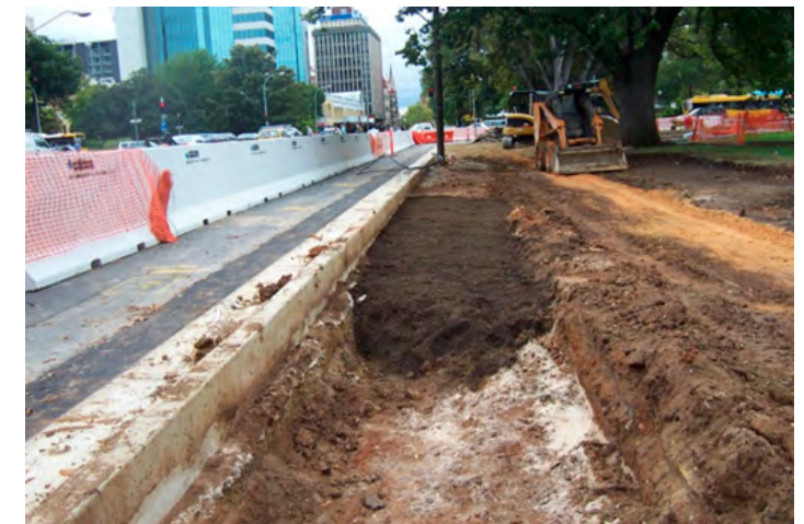
SPACE structural soil with 100% rooting volume being installed on Pulteney Street in Adelaide.
