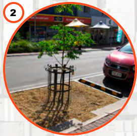
2 WSUD high soil volume tree pit with flush kerb enable passive irrigation from stormwater runoff
