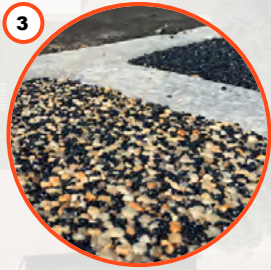
3 Permeable paver or Porous asphalt surface to the car park and footpath to improve tree health
