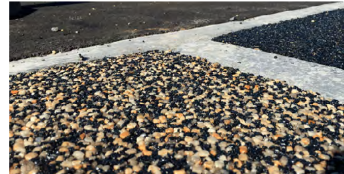
Laura Avenue, St Marys porous asphalt surface, City of Mitcham
