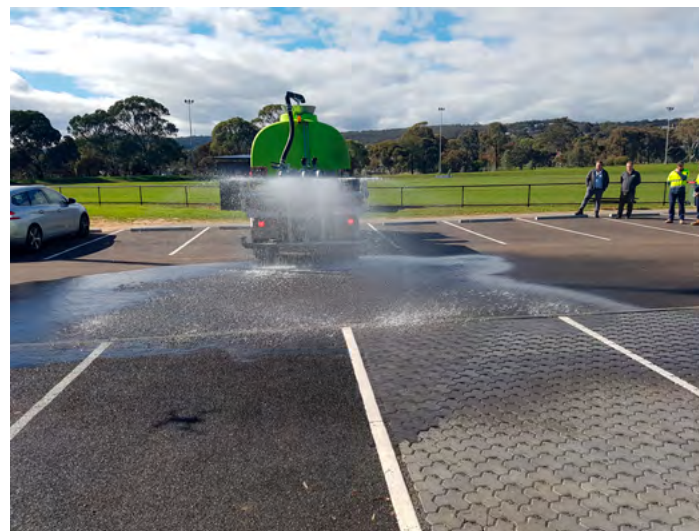
Laura Avenue, St Marys porous asphalt surface, City of Mitcham
