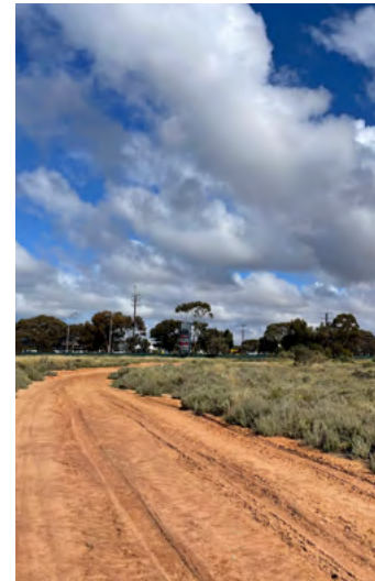
The unsealed roadway and the lack of vegetation cover on the levee have led to mud and soil erosion.
