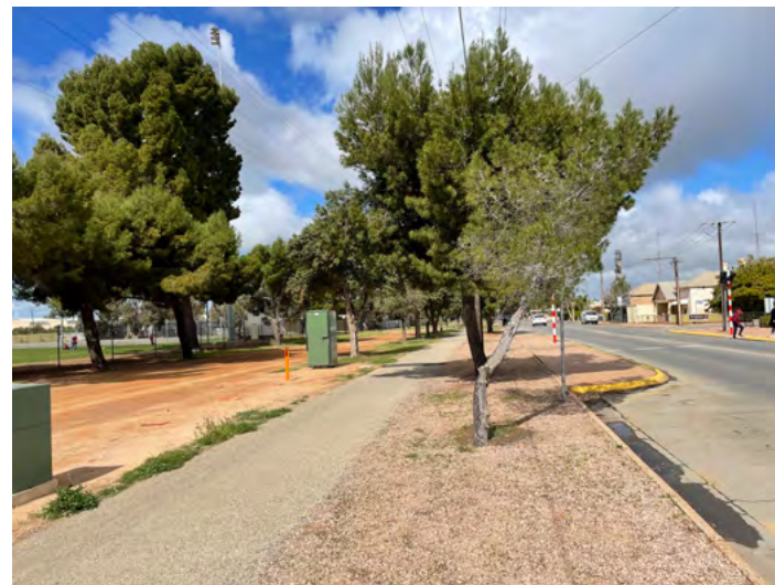
The footpath width is insufficient to meet the requirements of a shared path and will be widened.
