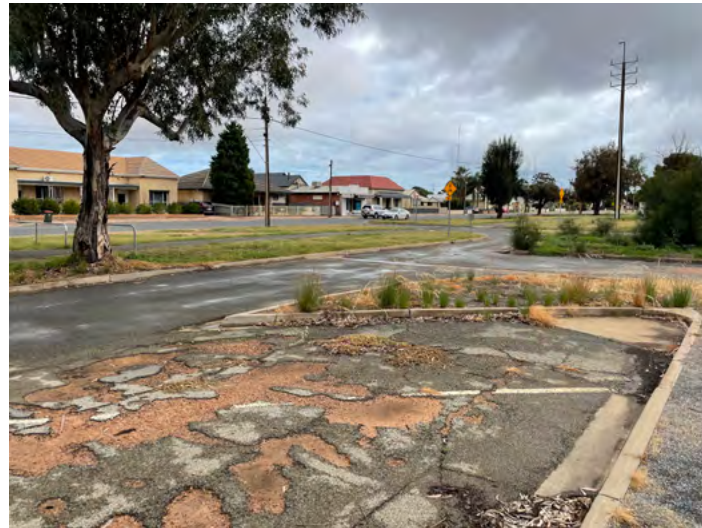
The western entrance of the park has a disorderly roadway, lacks pedestrian sidewalks, has poor visibility, and suffers from severe road surface damage.
