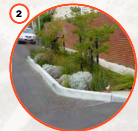
2 Adjustments to the car park traffic movement direction (optional) and upgraded bitumen + adding landscaped build-outs
