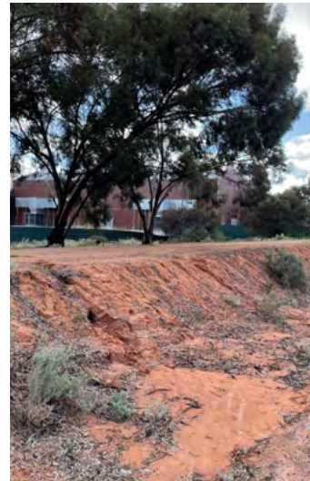
The unsealed roadway and the lack of vegetation cover on the levee have led to mud and soil erosion.
