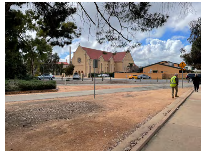
The main entrance of the park has exposed soil, and there is lack of pedestrian accessibility.
