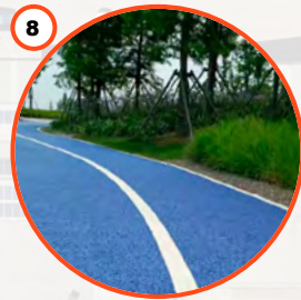
8 coloured bitumen surface secondary footpaths for improved accessibility and dust suppression
