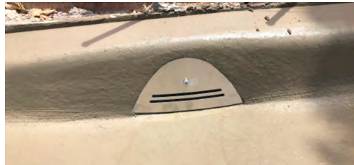
R750 kerb inlet (Treenet) more recent innovative approach to storage reservoirs, and has become widely adopted in SA and interstate.
