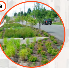
9 WSUD Infiltration trenches
