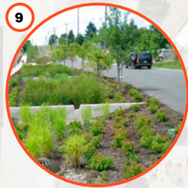
9 WSUD Infiltration trenches
