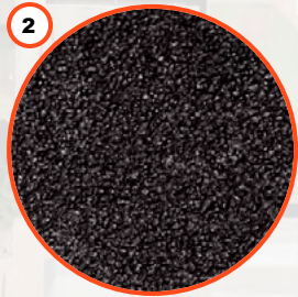
2 Spray seal / Asphalt surface carriageway.
