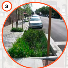
3 Build-outs with slotted kerbs to maximise passive irrigation opportunities
