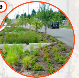
9 WSUD Infiltration trenches
