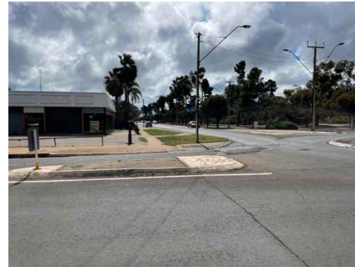
The roundabout lacks a pedestrian crossing, causing safety and accessibility concerns.
