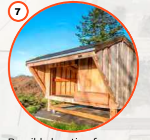
7 Possible location for a future birdwatching shelter.
