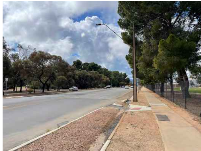
Very wide road reserve and wide carriageway.
