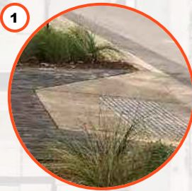
1 Formalised pedestrian crossing with pram ramps
