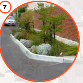
7 Formalised parallel car park with planted build-outs to maximise passive irrigation opportunities (optional)
