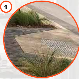
1 Formalised pedestrian crossing with pram ramps
