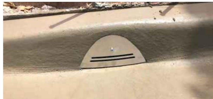
R750 kerb inlet (Treenet)
