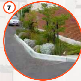
7 Formalised parallel car park with planted build-outs to maximise passive irrigation opportunities (optional)
