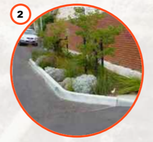
2 Adjustments to the car park traffic movement direction (optional) and upgraded bitumen + adding landscaped build-outs
