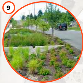
9 WSUD Infiltration trenches
