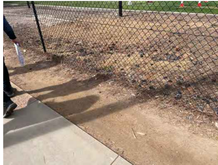
The soil on both sides of the footpath is exposed and lacks vegetation cover.
