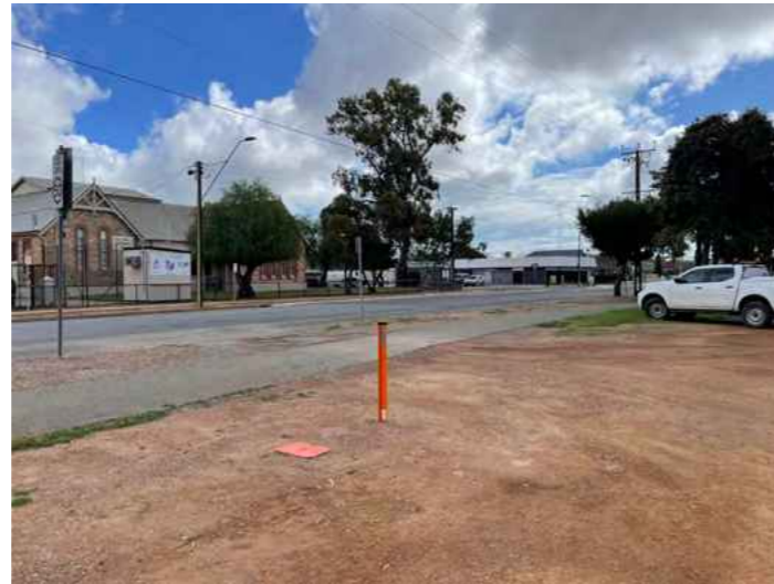
The informal entrance to the car park intersects with a footpath without clear signage, posing a safety hazard.
