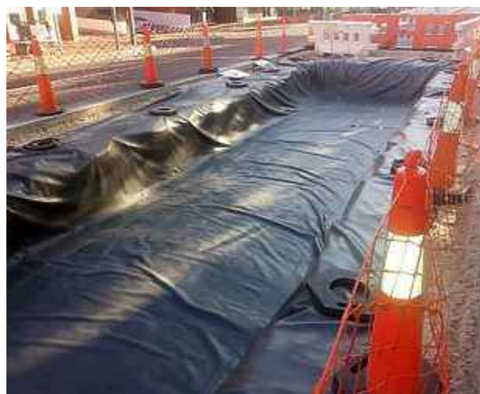
Poly membrane liner being laid at the base of tree pit to protect underground wastewater pipes.
