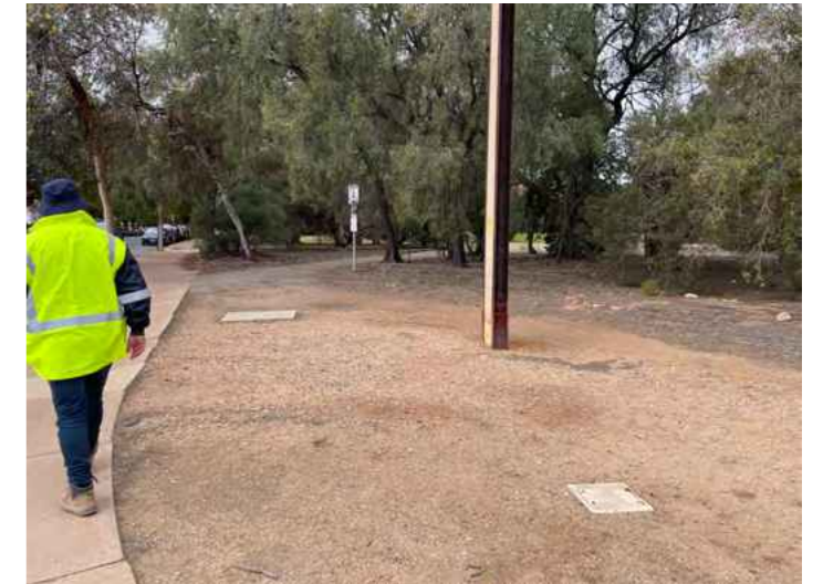
Angle new shared use path to connect up with path through reserve.
