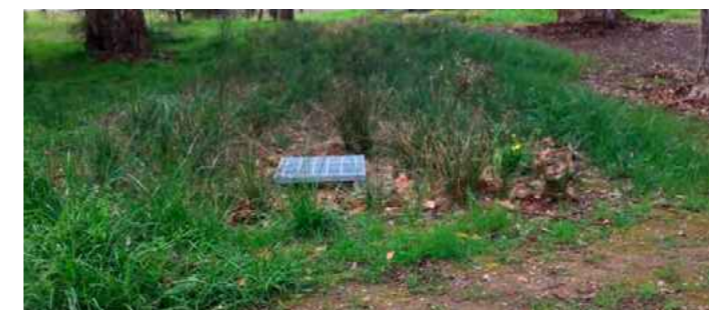
Park 18, Southern Parklands bioretention swale, Adelaide
