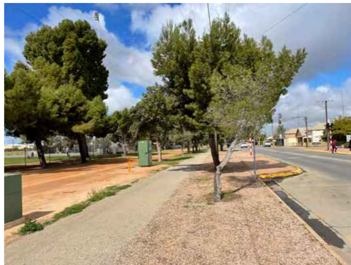
The footpath width is insufficient to meet the requirements of a shared path and will be widened.
