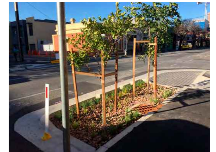
Raingarden/swales including lowered garden area for passive irrigation, and slotted kerbs allowing infiltration from roadway, on Wright Street in Adelaide
