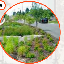
9 WSUD Infiltration trenches
