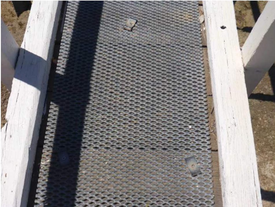
Photo 7 – Typical connections of steel grating to timber planks
