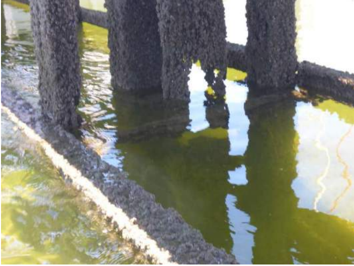
Photo 21 - Bent 19 deteriorated timber pile replaced with steel pile
