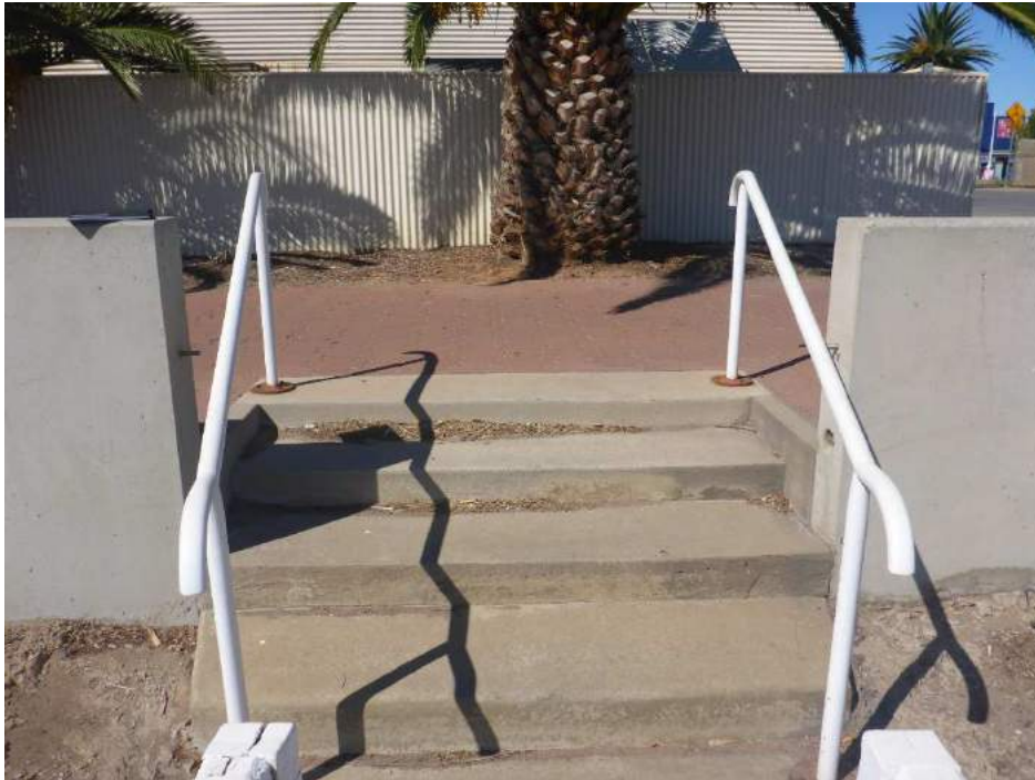
Photo 3 – Concrete stairs with room for ramp access to be provided
