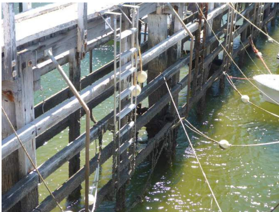
Photo 13 – Access ladders above water level at low tide
