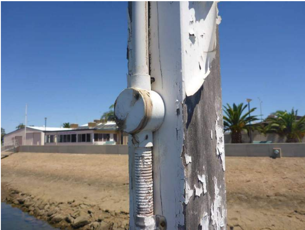
Photo 16 – Typical light pole installation
