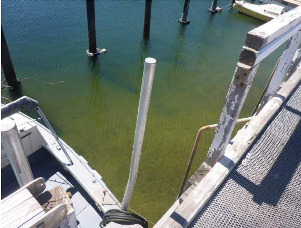
Photo 10 – Section of handrailing cut and hinged to form gateway for ladder access
