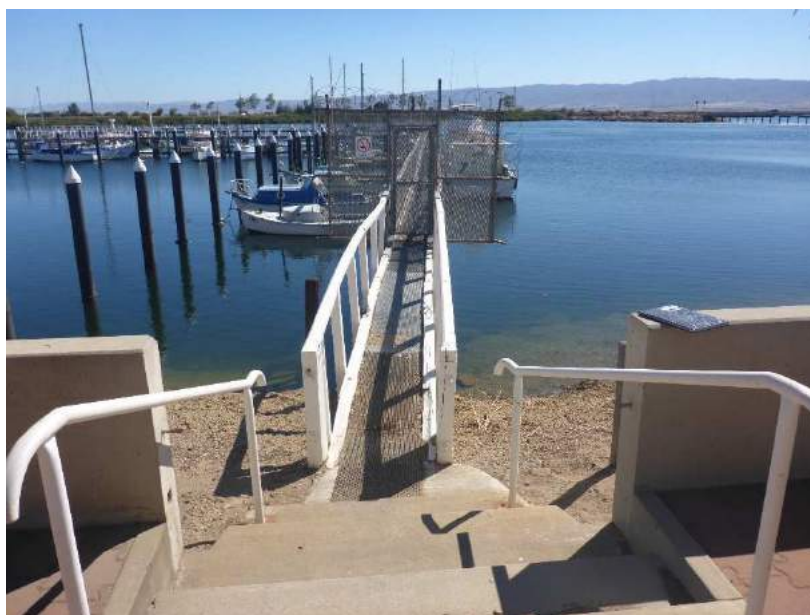
Photo 2 – Jetty approach with non standard concrete stairs
