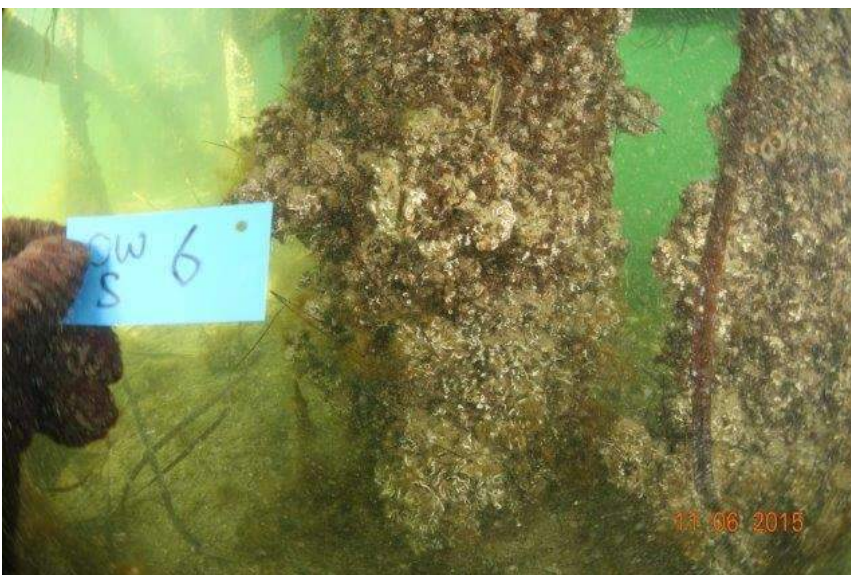
Pile condition at bent 6 south, outer walkway
