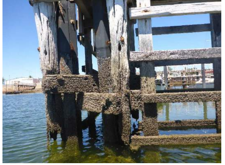
Photo 22 – Bent 21, end of main walkway replaced with 2 steel piles
