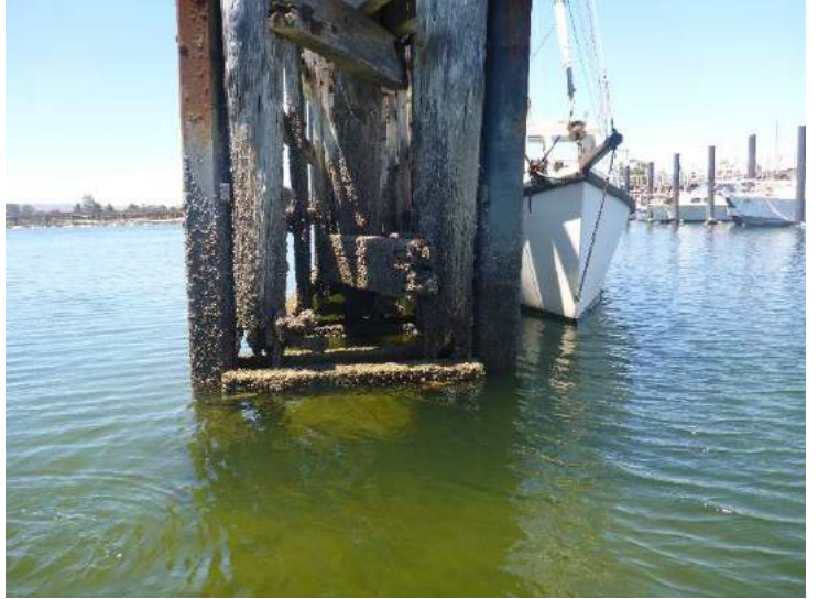
Photo 38 – Bent O12 (End)
