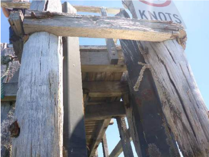
Photo 23 – Bent 21, steel replacement piles
