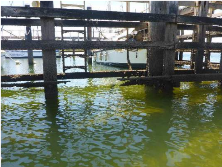
Photo 39 – Start of inner walkway, Bent I1
