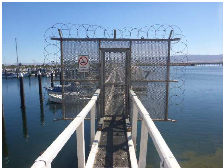
Photo 5 – Typical decking, kickboards and railing with security gate at start of jetty
