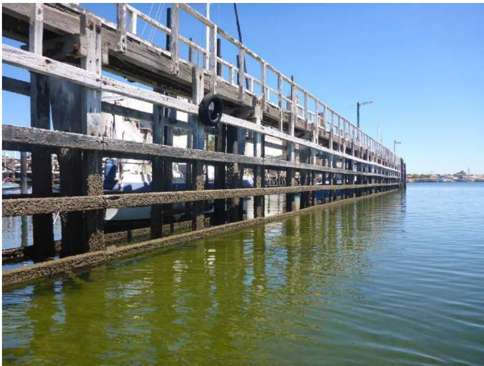
Photo 20 – Main set of piles with intermediate sets mid span between them
