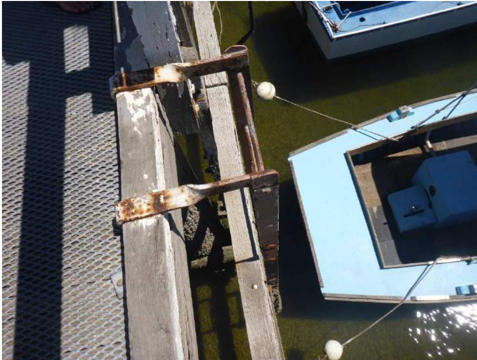
Photo 14 - Access ladder terminating at jetty deck level
