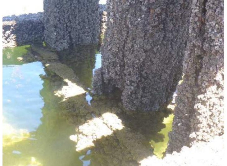
Photo 24 – Start of outer walkway, Bent O1
