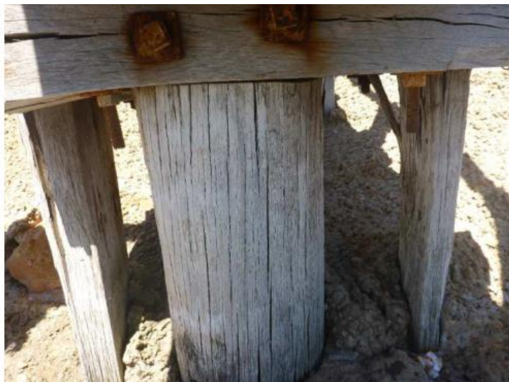
Photo 19 – Typical main set of pile layout with a central circular pile and two rectangular piles
